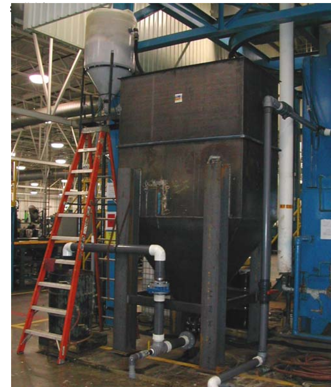
CLARIFLO Systems Tested On-site
